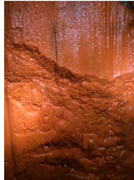
Same wall section cleaned using only low-pressure water through extended blowpipe nozzle
